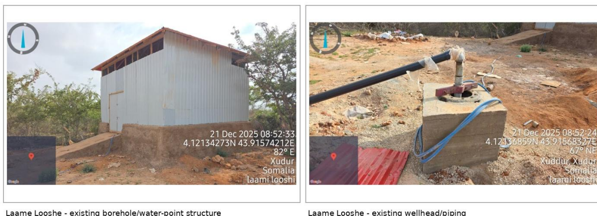
Figure 5-5: Representative Hudur Borehole Site / Existing Water-Point Condition
