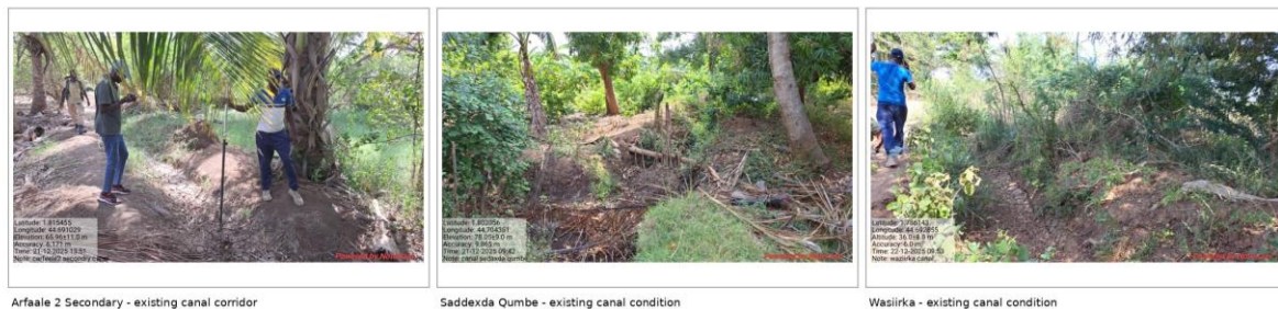
Figure 5-4: Representative Marka-Janale Canal Conditions Before Rehabilitation
