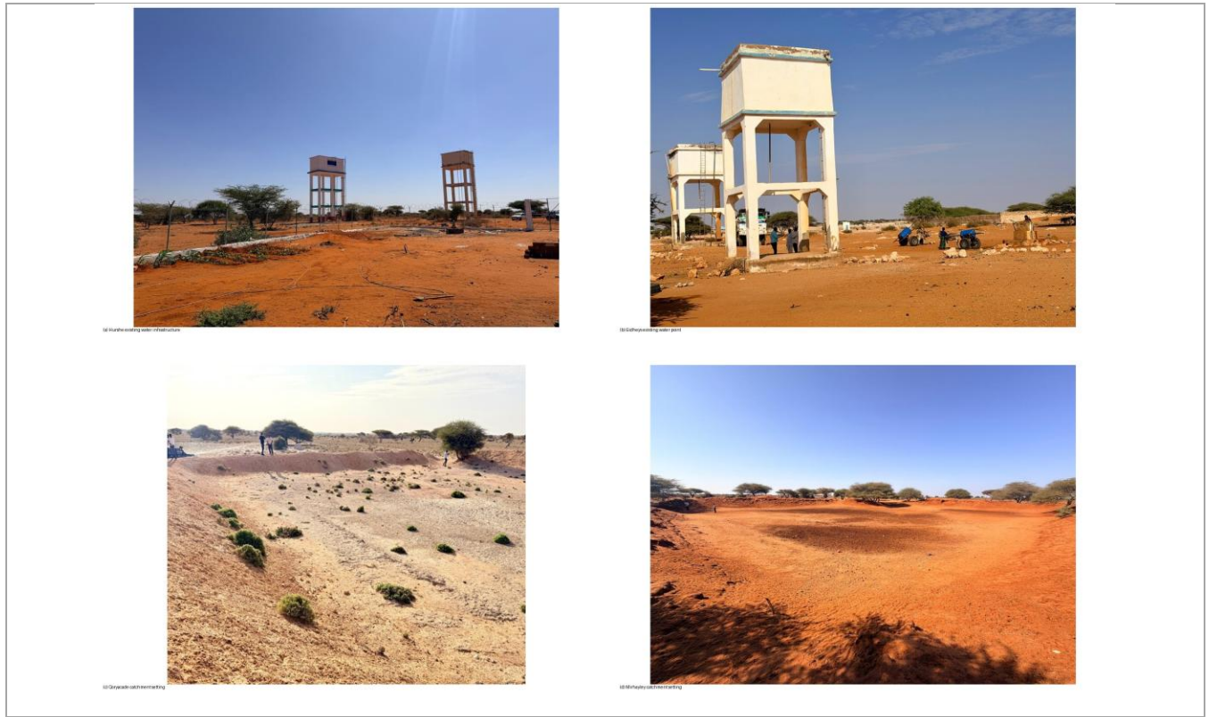
Figure 5-2: Representative Pre-Works Conditions - Borehole Infrastructure and Water Catchments in Galmudug
